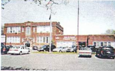
Existing conditions of the Town of Colonie Community Center, located within the Village of Colonie.
