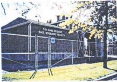
Salt Storage Facility
