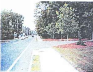
Sand Creek Road Sidewalk near Bauer Park
