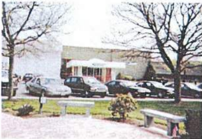
United States Post Office, across from the vacant Capital Plaza on Karner Road.
