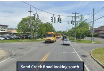
The southbound and northbound approaches on Sand Creek Road consist of a single 11-foot shared left/through/right lane. The eastbound and westbound approaches on Computer Drive South consist of a single 11-foot left/through/right lane. This intersection sees substantial peak-hour traffic due to adjacent commercial and office spaces. There is a marked crosswalk along the Computer Drive South westbound approach of the intersection in poor condition.
