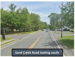
The southbound and northbound approaches on Sand Creek Road consist of one 11-foot lane in either direction. The Delafield Drive approach is stop-controlled and consists of a single 11-foot shared left/right turn lane. Delafield Drive is frequently utilized by residents and commuters as a connection to Central Avenue. There are no marked crosswalks at the intersection.
