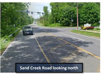
The southbound approach on Sand Creek Road consists of two 11-foot lanes, a through lane and a left turn only lane. The Shaker Run approach consists of two 12-foot lanes, a left turn only and a right turn only lane. The northbound approach on Sand Creek Road consists of two 11-foot lanes, a through lane and a right turn only lane. There are no marked crosswalks at the intersection.
