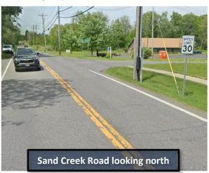
The southbound and northbound approaches on Sand Creek Road consist of one 11-foot lane in either direction. The South Family Drive approach is stop-controlled and consists of one 11-foot shared left/right turn lane. There are no marked crosswalks at the intersection.
