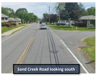
The southbound and northbound approaches on Sand Creek Road consist of one 11-foot lane in either direction. The Myers Court approach is stop-controlled and consists of a single 11-foot shared left/right turn lane. There are no marked crosswalks at the intersection.
