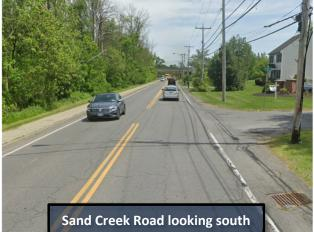
The southbound and northbound approaches on Sand Creek Road consist of one 11-foot lane in either direction. The Jo Ann Court approach is stop-controlled and consists of a single 11-foot shared left/right turn lane. There are no marked crosswalks at the intersection.
