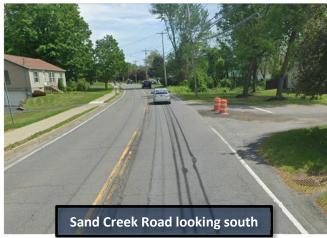
The southbound and northbound approaches on Sand Creek Road consist of one 11-foot lane in either direction. The Terry Court approach is stop-controlled and consists of a single 11-foot shared left/right turn lane. There are no marked crosswalks at the intersection.
