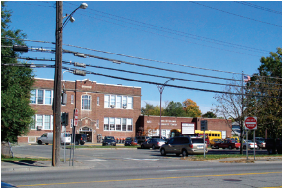
The center of the Community Center facade projects, and has a raised roofline to break up the massing and accentuate the entrance.
