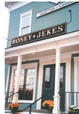
Successful transition of residence to commercial storefront.
