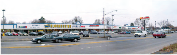
An example of a typical upstate strip mall (Rome, NY). Negligible site improvements or attempts at creating beautiful neighborhood character have been made.
