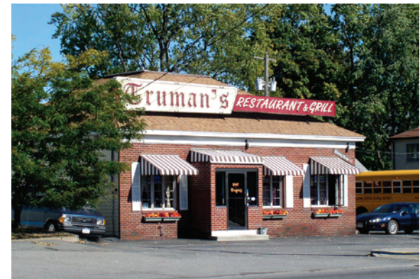
Signs can add character to the district, and should be part of an overall facade design.
