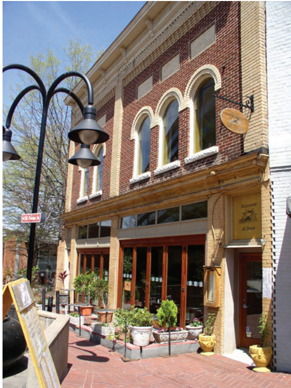
The first floor "windows" are actually doors that pivot and slide, opening the first floor completely to outdoor seating.
