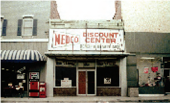
Signs should not cover historic detailing of upper facade. Overall untidy designs and lack of maintenance detract from a building's professional appearance. Courtesy of National Trust for Historic Preservation.
