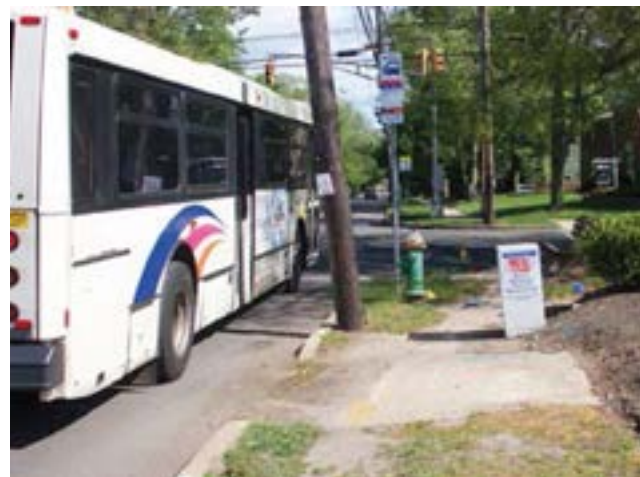
The bus stop above lacks an ADA-compliant landing-pad and sidewalk connection.
