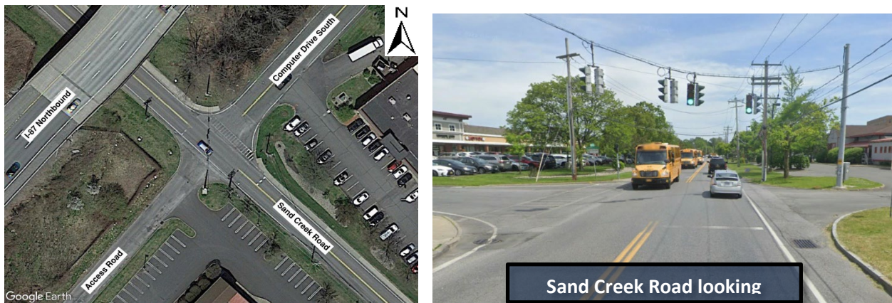
Figure 2.17: Sand Creek Road and Computer Drive South Intersection
