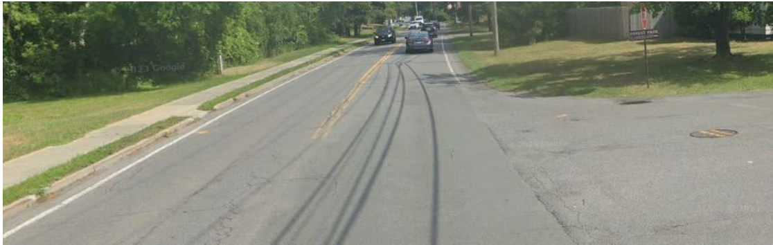
Figure 5.8: Sand Creek Road looking south at Mordella Road
