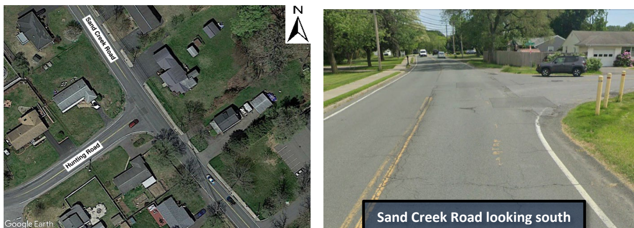
Figure 2.7: Sand Creek Road and Hunting Road Intersection
