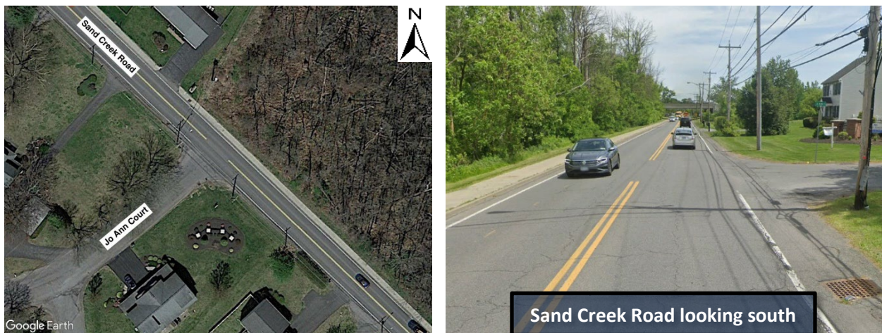
Figure 2.15: Sand Creek Road and Jo Ann Court Intersection
